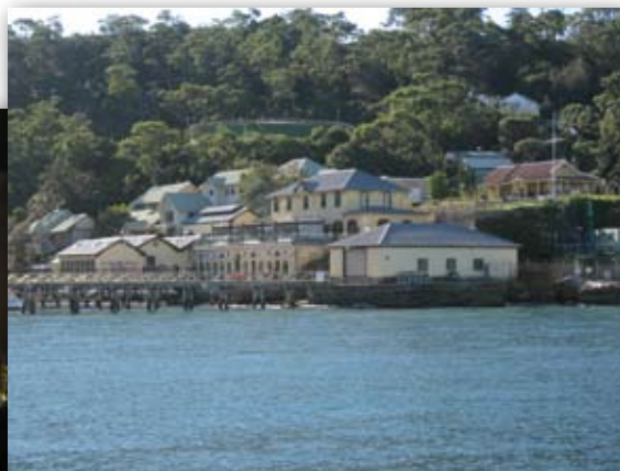
Figure 3. The Sydney Institute of Marine Science (SIMS), a not-for-profit marine research facility, was established in 2005 by four of Sydney's leading universities.
